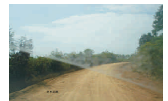
修缮后的乡村公路 After the renovation of the rural roadway
