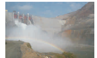
泄洪中的班查电站大坝 Release flood waters, BAN CHAT dam
