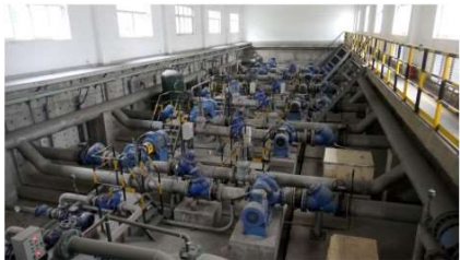
Construction of circulating pump house (industrial cooling)
